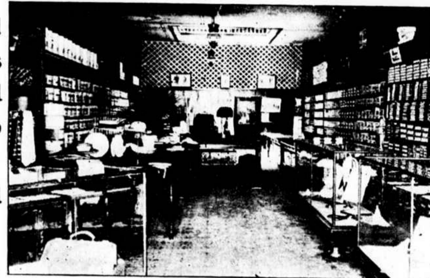
Interior view of Bomar & Crigler's
