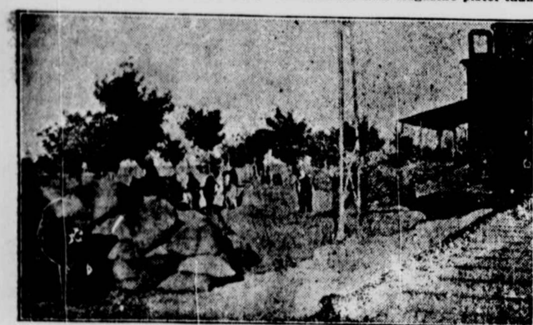
Shoveling Grain on the Line of the Bagdad Railway.
