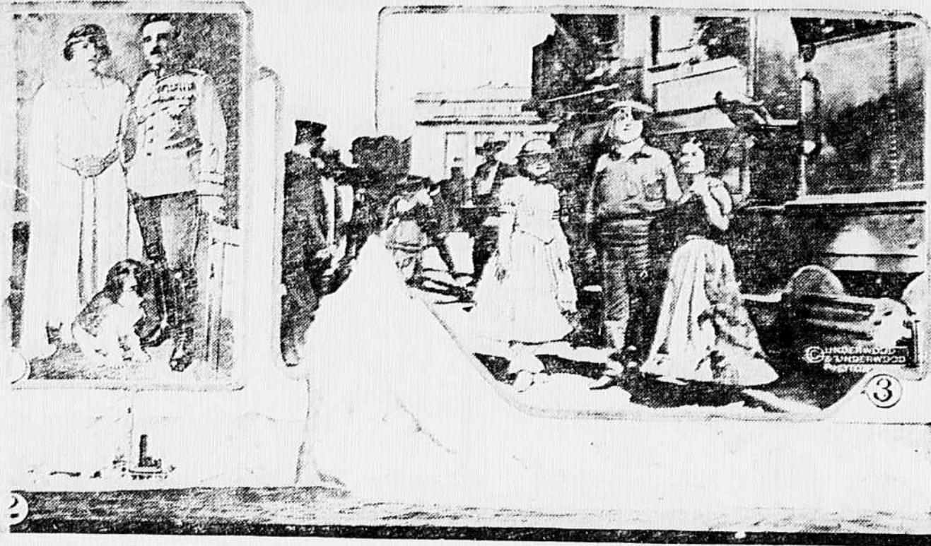
—Official photograph of the first steamer of the North American coast, illustrating work of those who are in charge of the construction of the Panama Canal. —California's first locomotive and its engineer, J. L. ...
