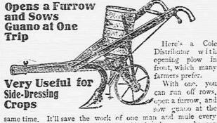
Distributor with opening plow in front, which many farmers prefer. With one, you can run off rows. open a furrow, and sow guano at the planting day. Especially good for side-dressing-can be run
