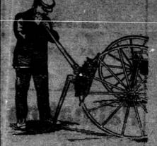
I have the Schan Cold Tire Setter. Tires are Tightened Cold, without removing whell: M. S GUNTER
