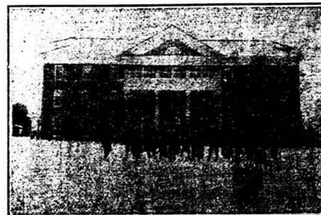
GUILDS HALL, CARLISLE SCHOOL
