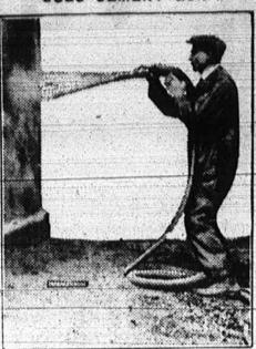
Houses are being erected in Southend, England, with the aid of a cement gun. A frame of timber is bolted together with expanded metal, onto which is pumped by a 60 horse power motor a substantial thickness of sand and cement. This is the first building constructed in this manner in Eu-
