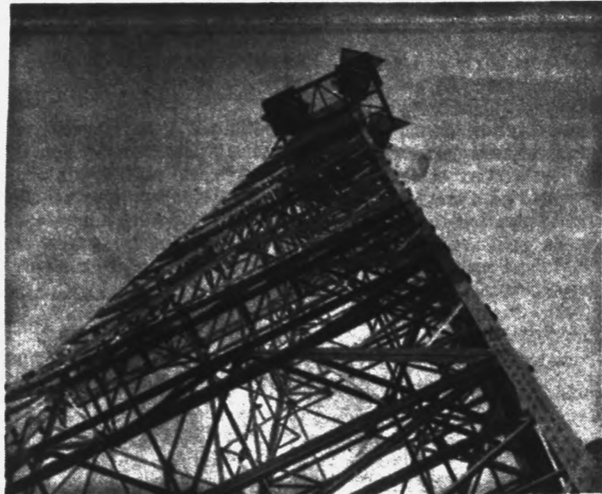
GROUND VIEW OF TELEPHONE TOWER
