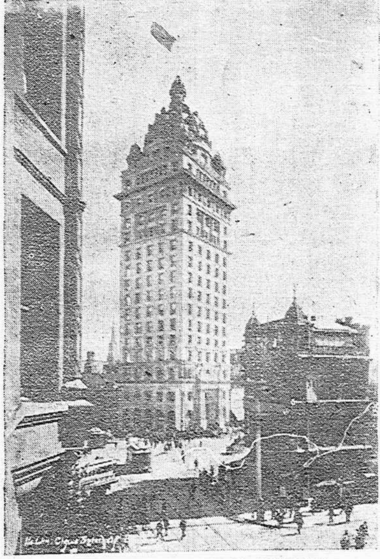
THE CALL BUILDING, ALSO DESTROYED.
