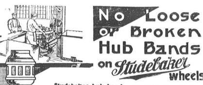
Studebaker hub bands are made of a specially refined iron perfectly adapted for this use. Hub bands are welded by electricity and then shrunk on by hydraultc pressure.
