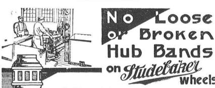
Studebaker hub bands are made of a specially refined iron perfectly adapted for this use. Hub bands are welded by electricity and then shrunk on by hydraulic pressure.
