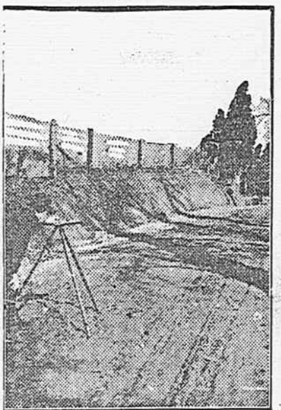
Getting Road Levels Preparatory to Improving Highways.
