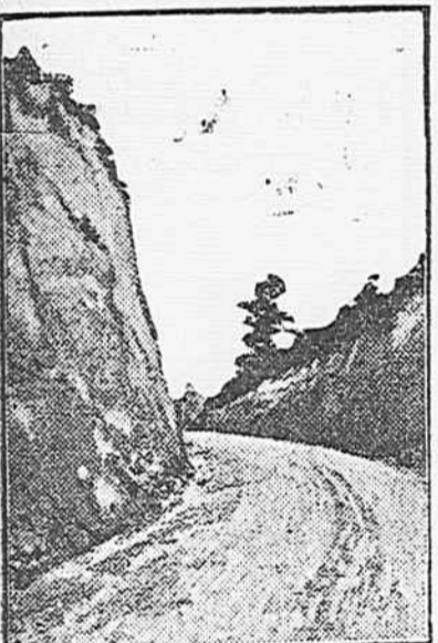
Cut Through Mine Hole Gap in Asheville-Charlotte Highway.
