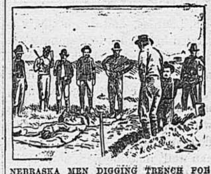
NEBRASKA MEN DIGGING TRENCH FOR THE BURIAL OF DEAD FILIPINOS.
