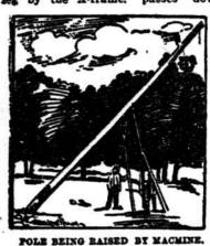
around the sheave at the lower end of the pike pole, and up over a similar sheave near the upper end of the righthand end of the A-frame, whence it soes to a winch or "crab" mounted on the frame. It is obvious that turning the handle of the crab in the proper direction will wind up the rope or cable on the drum and raise the telescoping pike.
