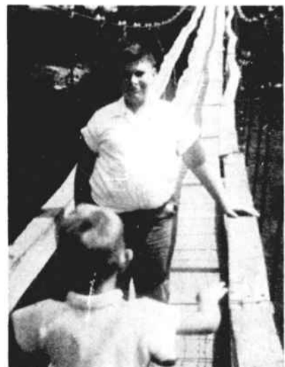
TOMMY , son of the Freeman Lanfords, Clinton Mills, is shown standing on a swinging bridge at Cherokee, N. C. The next day the bridge collapsed, killing two and injuring many others. Close shave for Tommy.
