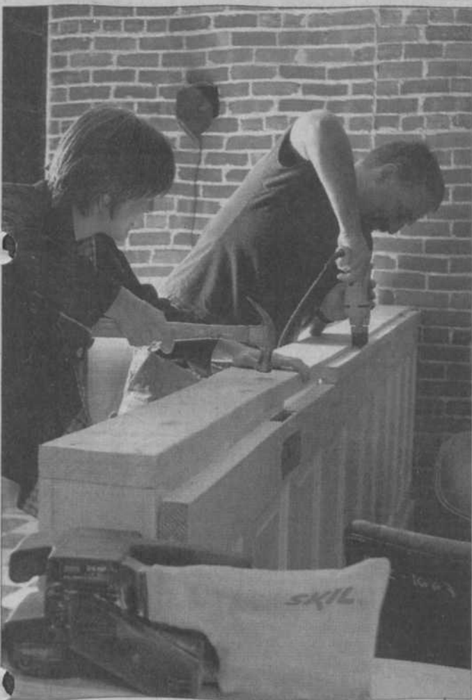
PHOTO BY MORGAN FORD/THE GAMECOCK Marianne Parrish and Bill Florian work on construction at the Red Tub Bar, which they plan to open by midsummer.
