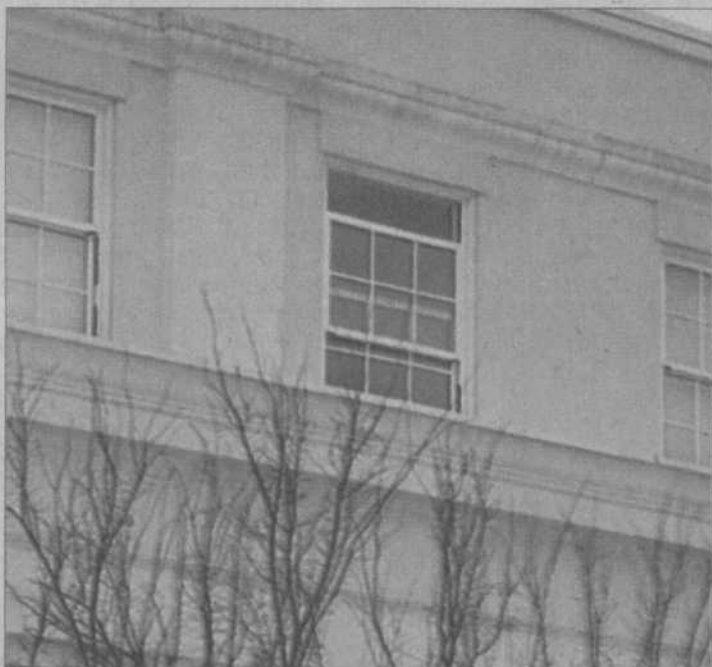
A smoke bomb in the southwest stairwell of South Quad filled three floors of the building with smoke.
