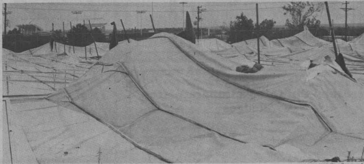
The Bubble, USC's air-inflated indoor sports facility, was destroyed when Hurricane Hugo hit Columbia Thursday night.
