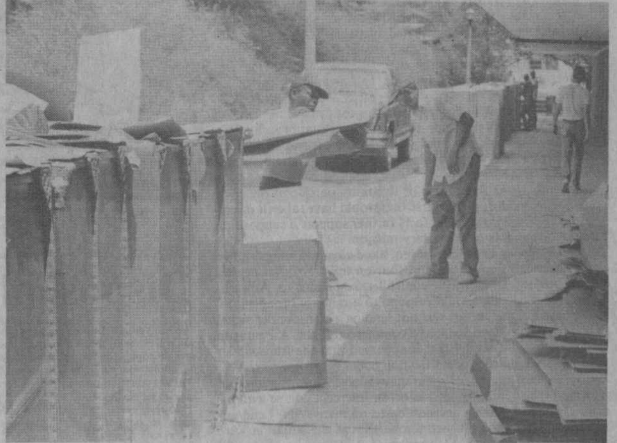
Dorm renovations outside the Towers area. New furniture is being unloaded for the dorms.
