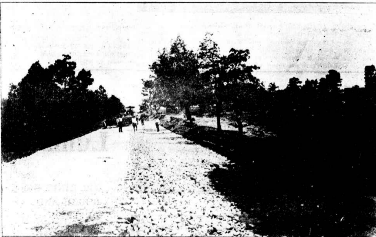
ROAD BEING GRAD.
