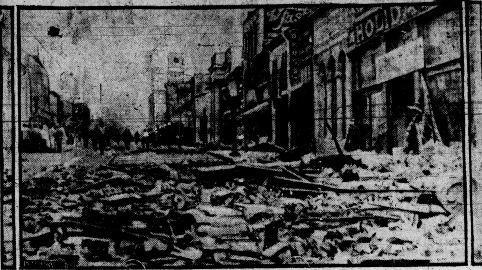
These pictures, transmitted by American Telegraph and Telephone wires, show the ruins on State street, the main business thoroughfare of Santa Barbara, immediately after the earthquake.
