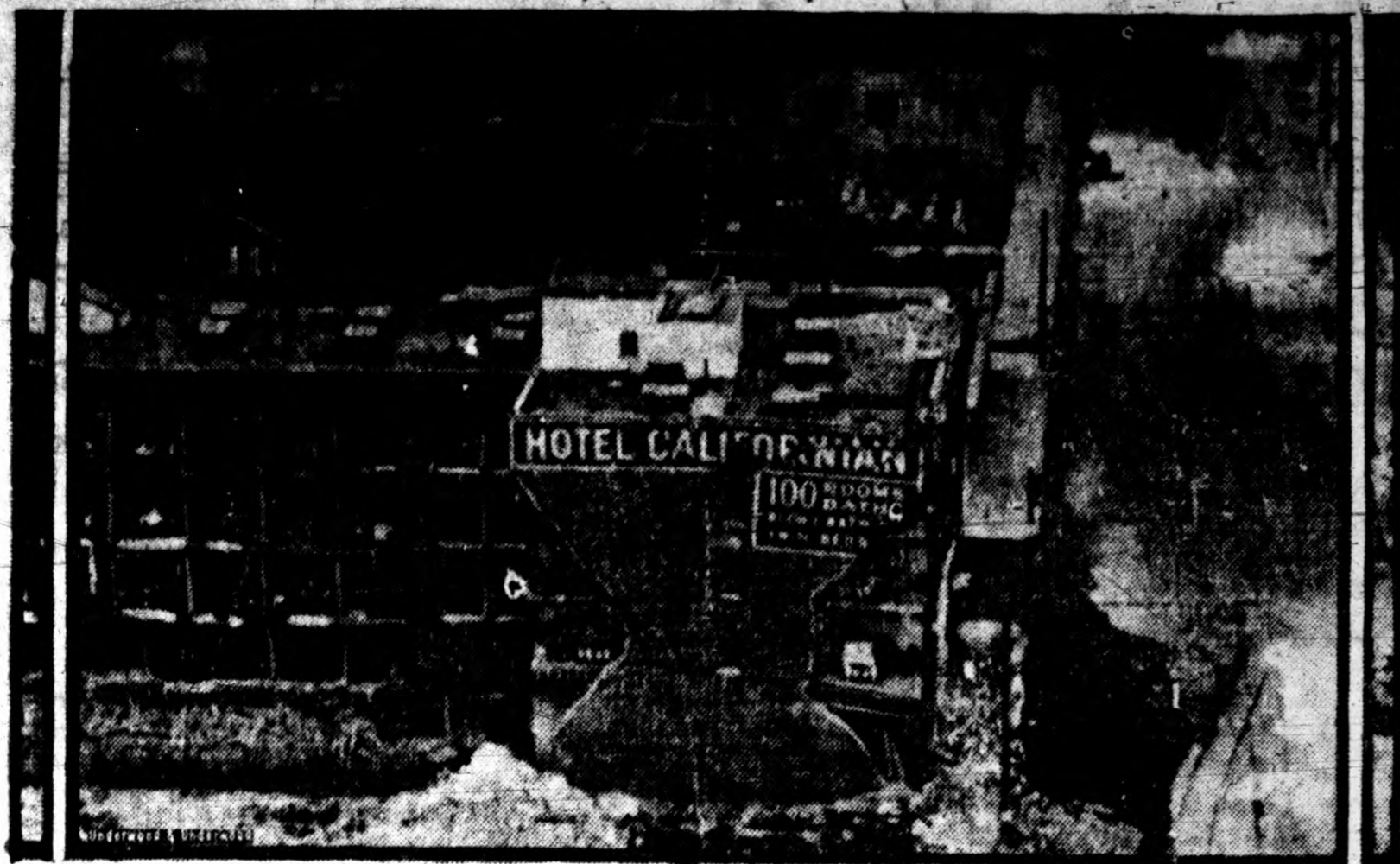
This remarkable picture, received over the wires of the American Telegraph and Telephone company, was taken during the earthquake that wrecked Santa Barbara, Cal., and shows the ruins of the Hotel Californian and other buildings on State street.
