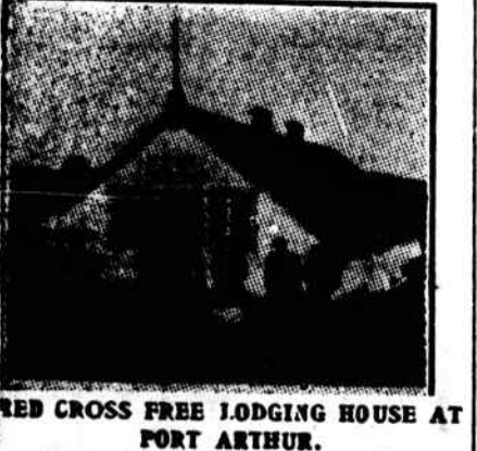
FREE LODGING HOUSE AT PORT ARTHUR.
