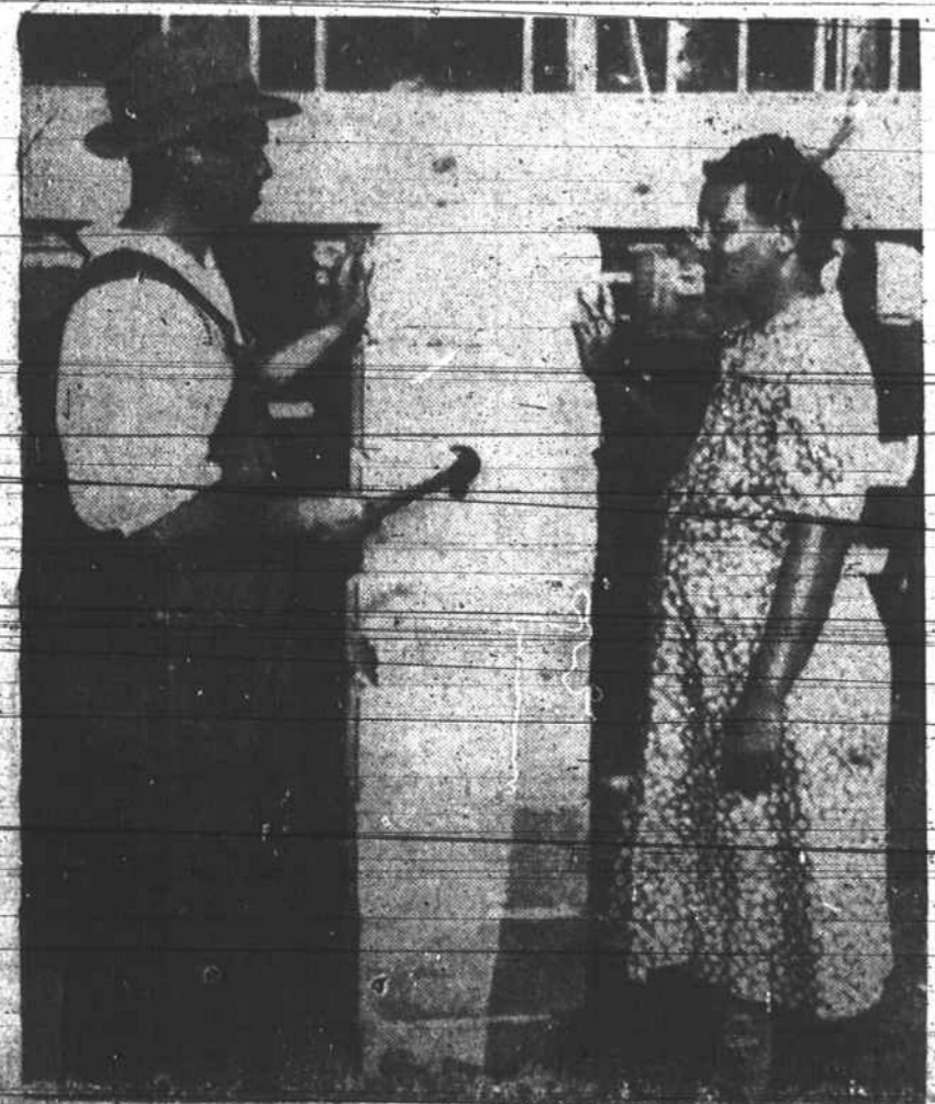
TALKING OVER CONSTRUCTION WORKERS' HITS, Paul Stevens appears optimistic over construction progress on the temporary home that is being built for her and her seven children through the cooperation of the Atlanta Chapter Red Cross and interested citizens. She talks over construction with Charlie Ray, the supervisor at the Rockdale Park location. The Stevens family was forced to live in the basement of a funeral home before their plight came to the attention of citizens and Red Cross authorities. (Photo By Perry)
