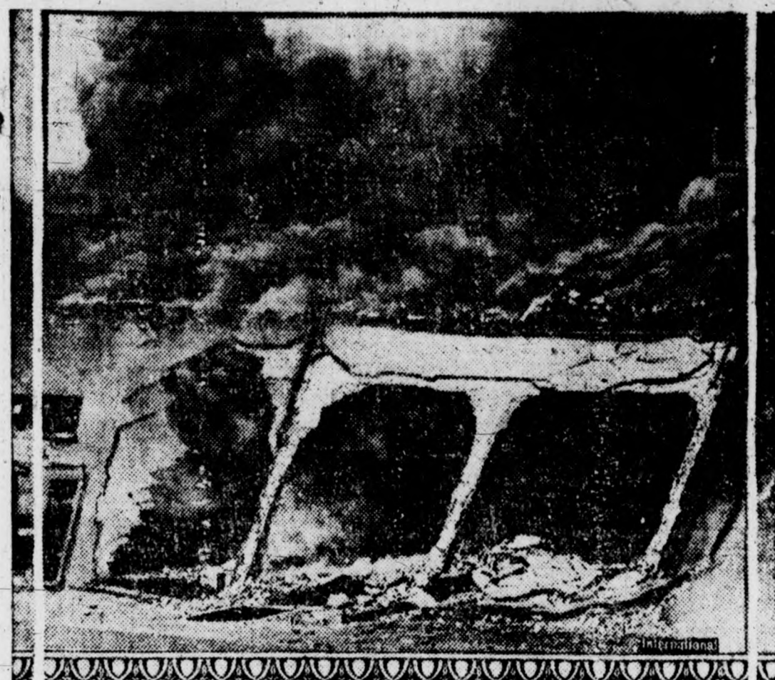
The scene of the spectacular fire which destroyed the Terminal building Toledo's principal public auditorium. The fire was of undetermined origin, and within half an hour after it started the entire structure was in flames. The loss was $200,000.
