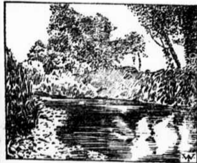
UNLINED CANAL. (Showing vegetation.)
