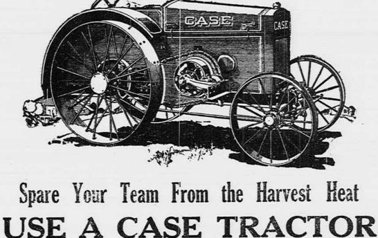
Make this season your mo t profitable one by getting a Case Tractor to do your harvesting With a Case 9-18 Tractor you can pull any size binder. Under favorable conditions it will handle two 6-ft. binders (r ght or left hard cut). The Case 10-20 Tractor will handle two 7-ft. binders under ordinary field and soil conditions. Larger Case Tractors will successfully pull more units proportionally.
