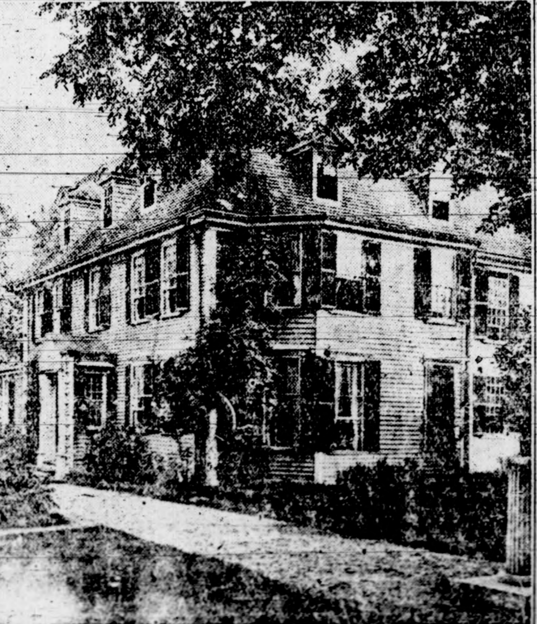
QUINCY, MASS., BUILT IN 1685. Quincy's classic example of a clapboard building preserved for over two hundred years by careful and frequent painting. It has secret panels, chimney, air-escape and being places, said to have been used by smugglers. Later the home of great statesmen and of the famous belle, Dorothy Quincy.
