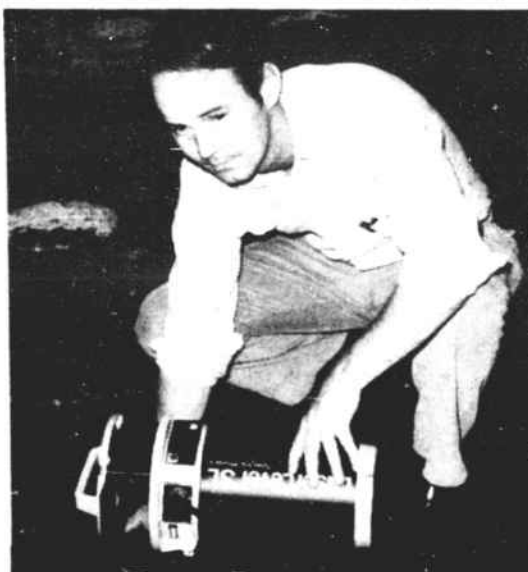
LASER BEAMS USED TO LINE AND LEVEL WEAVING MACHINES —Mechanical Engineer, Harry Sullivan, utilizes a Laserlevel to lay off floor at Bailey for new Sulzer Weaving Machines.
