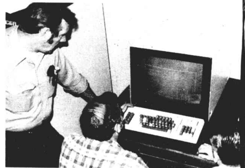
REVIEWING TRANE CONTROLS —Gerald Satterfield, Toland Snelgrove and Plants 1 and 2 Engineer Arthur Sanders review the new Trane Sentinel refrigeration controls.
