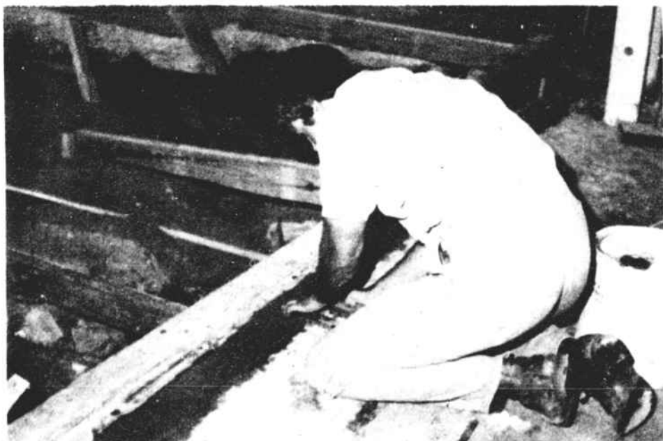
Contractors preparing slasher doffer pit.
