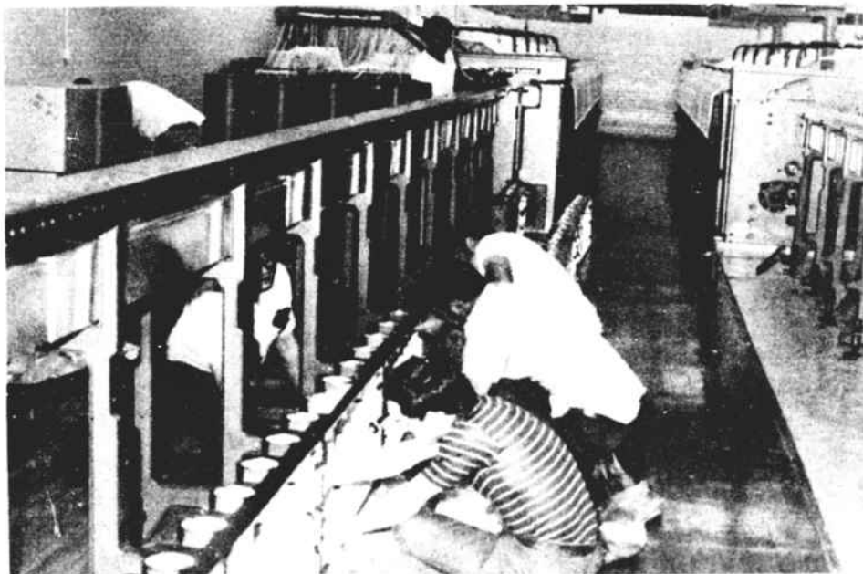
Technicians are carefully assembling new Saco-Lowell roving frames.
