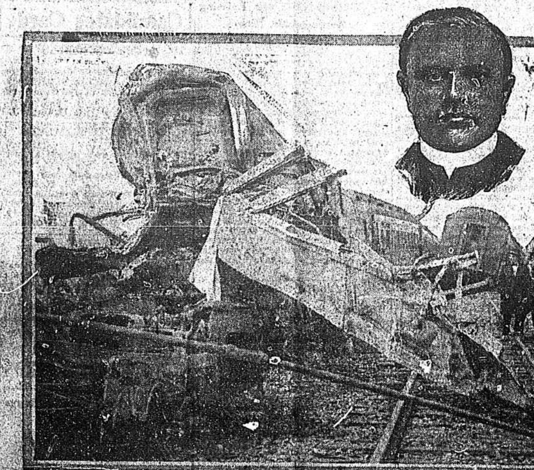
The "death car" in the New York Central wreck at Amherst, Ohio, is beneath the locomotive shown in this photograph. That is, what is left of the trucks are beneath the locomotive. Part of the vestibule of the car in which so many persons lost their lives clings to the forward part of the engine. The locomotive hauled the second section of Train No. 88. The picture also shows the Rev. Gustav Valpi, the Detroit clergyman, who was killed in the wreck.
