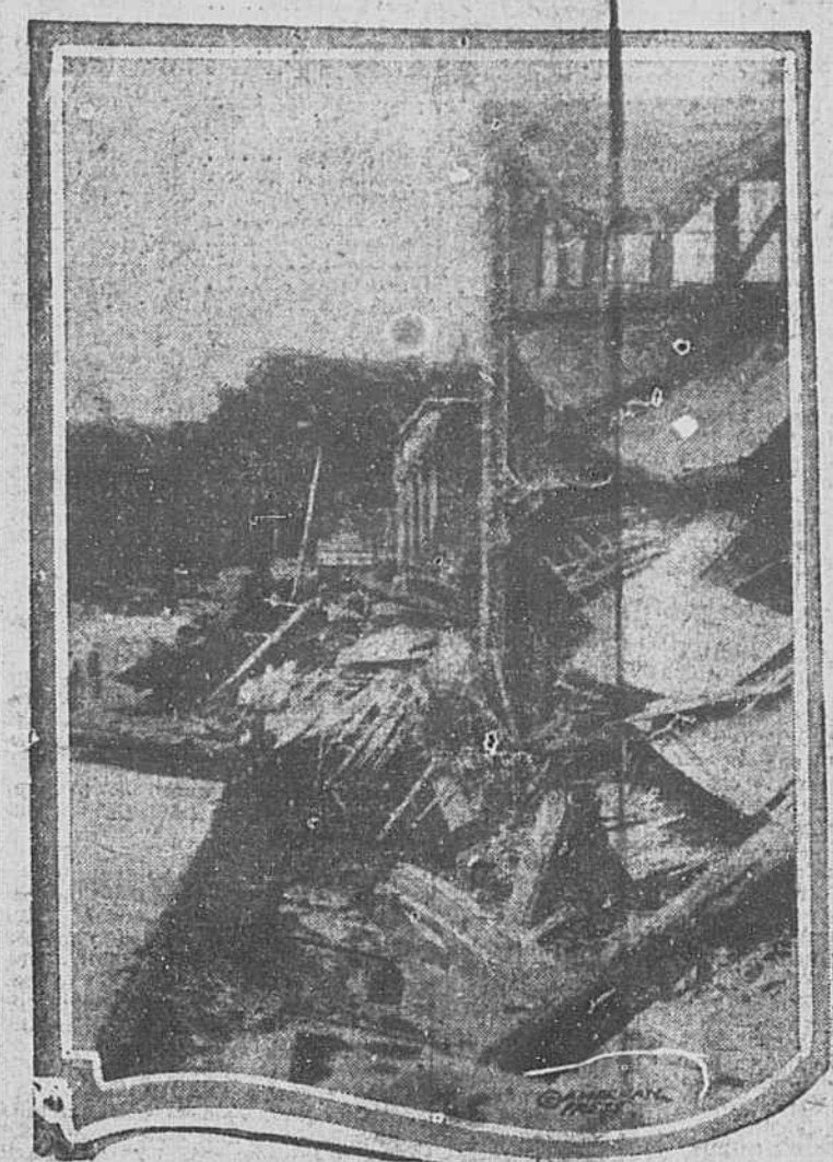
More than forty persons were killed and more injured in the storm and flood which swept through Erie, Pa., Tuesday, Aug. 3.—This photograph shows the damage done one building. Many more were left in the same condition.
